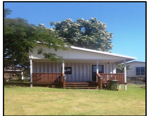
Figure 20: NUSSA Container Office
