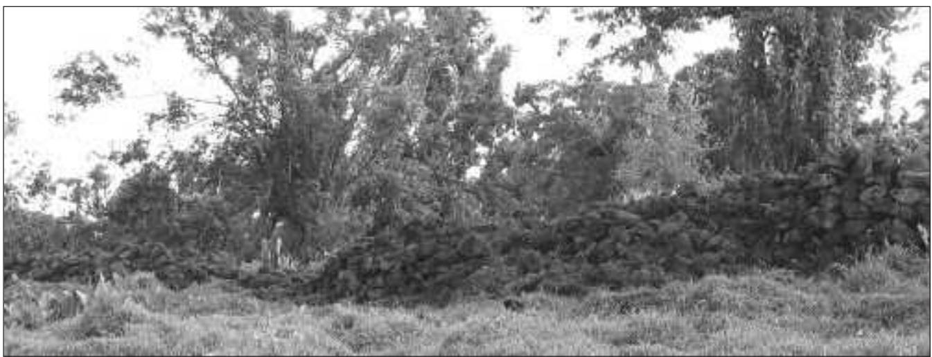
Figure 22. Part of the cleared Pa Tonga wall. (Photo Helene Martinsson-Wallin)
